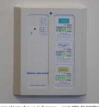
Area alarm shown is 3 gases - part #PX-DUXXOVA
